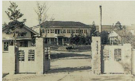
Entrance of Factory (1939)
